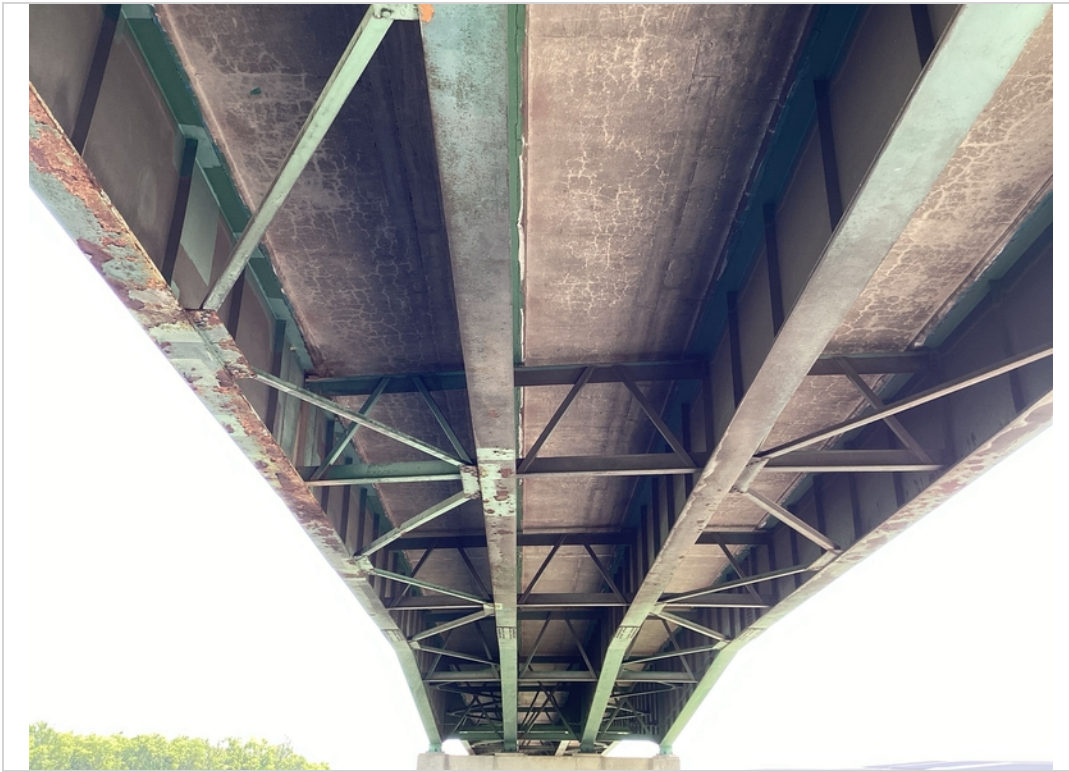
Bottom of Deck Span 2
