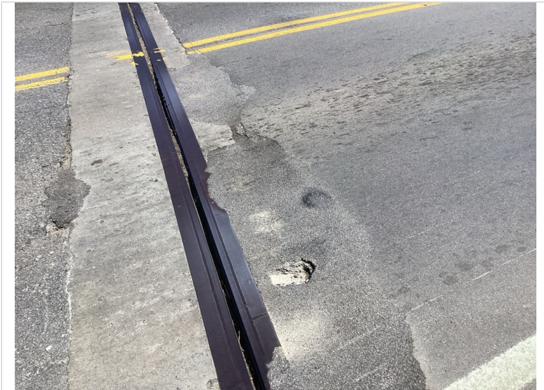
A approach pavement A/C patches
