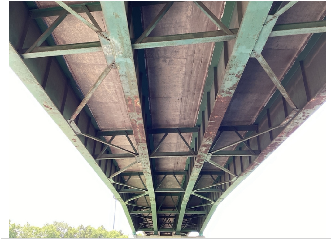
Bottom of Deck Span 1
