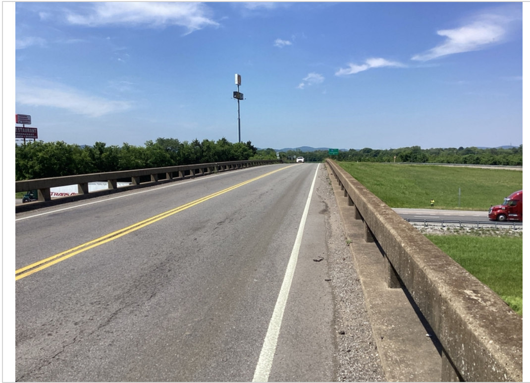
View along deck
