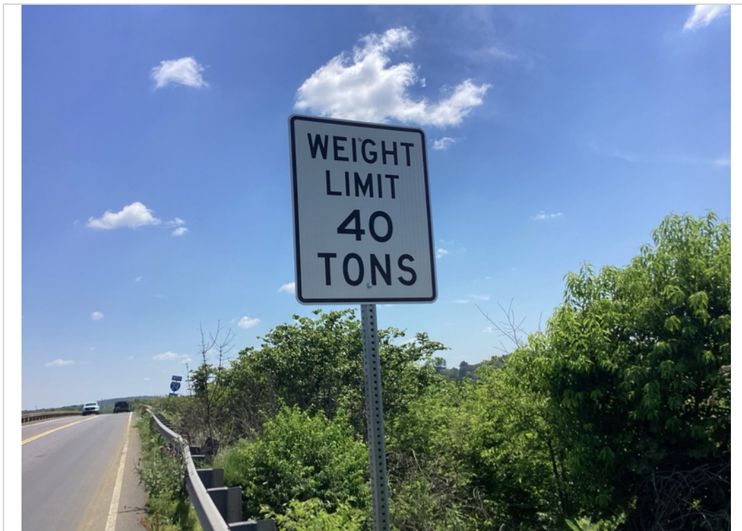
B approach weight posted sign
